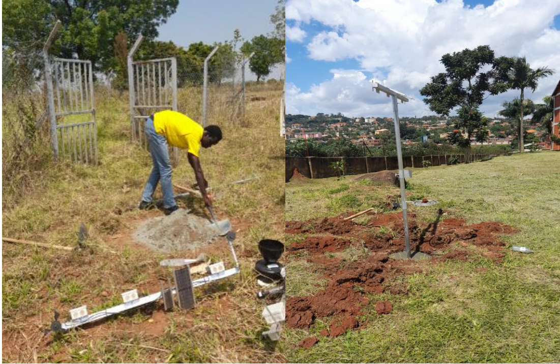
Figure 4.3: Making the concrete base and fixing the stand
