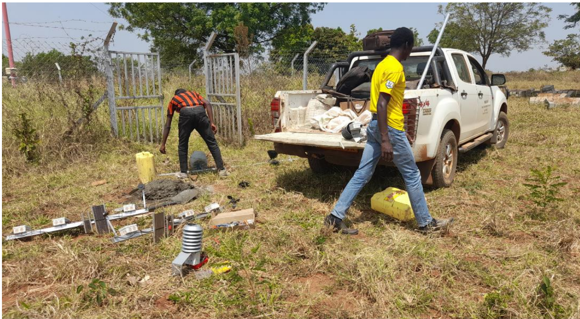
Figure 4.2: Making the concrete for fixing the stand
